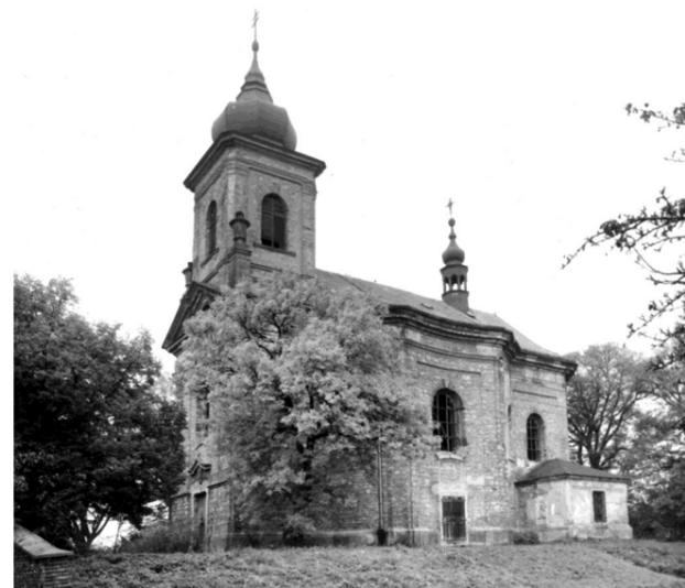
changing water conditions around the church resulting in moisture wicking into its walls and causing such severe stability problems that part of the nave's vaults collapsed. As a result of these problems, the church was closed in 1951 and then fell into disrepair.
