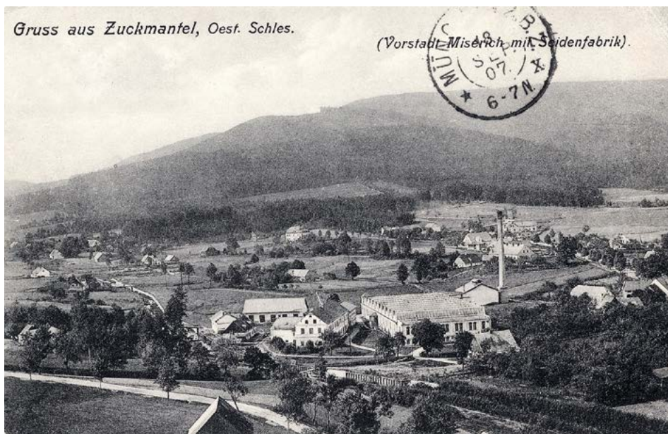
Zlaté Hory, J. Adensamer & Co. silk goods factory, early 20th century. The left part of the site, bordering on the Zlatý Potok stream, consists of the buildings of a former paper mill. At the right is the weaving mill hall with the adjacent boiler house and chimney. Městské muzeum ve Zlatých Horách (Zlaté Hory Municipal Museum).
