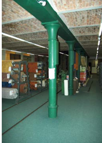
Šumperk, K. Siegl sen. mechanical weaving mill, building containing auxiliary and preparatory shops, 1889, cast iron columns in the basement and on the second floor and original building, 1860, and warehouse, offices, 1880. Photograph by Michaela Ryšková, 2006 a 2021.
