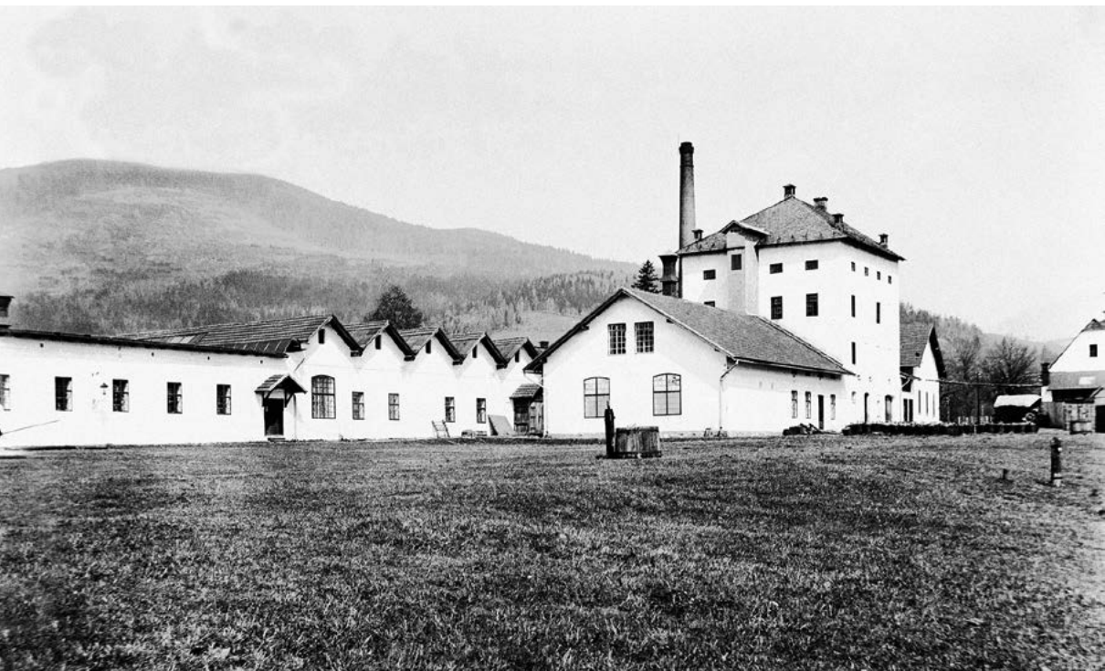
Loučná nad Desnou, Rejhotice, G. Ulrich bleaching shop, turn of the 20th century. From the left the mangle, beetling mill and calender shop (in the building with the sawtooth roof), in the foreground the single-floor starching shop with a gable roof, in the background the winter drying house and an administrative building. Photograph by Gustav Ulrich, collection of the Rolleder museum association (Muzejní spolek Rolleder), Odry.
