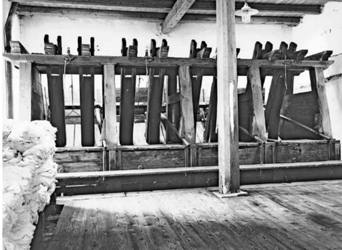
Loučná nad Desnou, municipal subdivision Rejhotice, G. Ulrich, linen goods bleaching and finishing plant, photographs from the late 19th/early 20th century. Hammer beetling mill (top), bleachery with soaking vats, fabric boiler and draining mangles (centre), hydraulic mangle (bottom). Photograph by Gustav Ulrich, Rolleder museum association, Odry,
