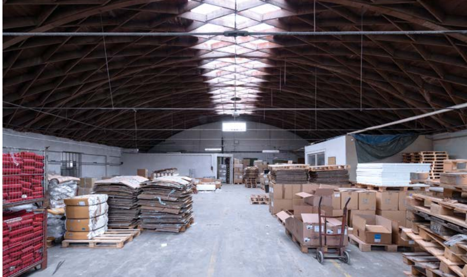
Šumperk, Vinciguerra & Cie. thread spinning mill, factory hall (1930) with lamellar ceiling. Photograph by Viktor Mácha, 2019.
