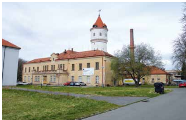
Fig. 4.195: Prague-Bohnice (Psychiatric Hospital Bohnice) – washhouse block No. 25. The extensive complex of the psychiatric hospital was created from 1905 to the 1930s. The author of most of the buildings, Václav Roštlapil, also designed an elevated water tank from 1908. Cold non-potable water was pumped into the tank on the top floor; below it there were two expansion tanks for regulating the pressure of the heating system; lower there was a hot water tank and further lower a tank for lukewarm water which led to the bath. Cold water flowed gravitationally downwards where it was heated by steam and it ascended by itself to the hot water tank from where it was distributed gravitationally to the complex. The waterworks was used until 1972. The original petrol station building was rebuilt into an apartment unit. Photograph by Michaela Ryšková, 2022.
