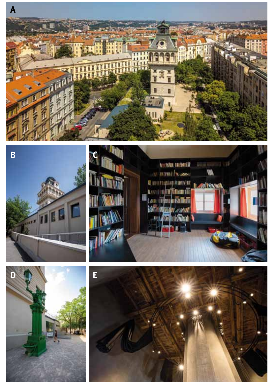
Fig. 5.21: Prague-Letná – elevated water tank, conversion: (A) overall view; (B) wheelchair accessible entrance; (C) library; (D) cast-iron water pillar fountain with a minimalist extension; (E) chimney passing through the centre of the water tank. Photograph from the National Heritage Institute archive.
