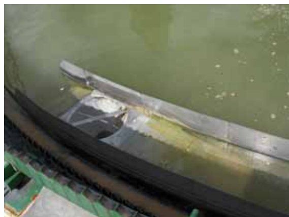
Fig. 4.245: Overflow edge. Photograph from the TGM WRI archive.
