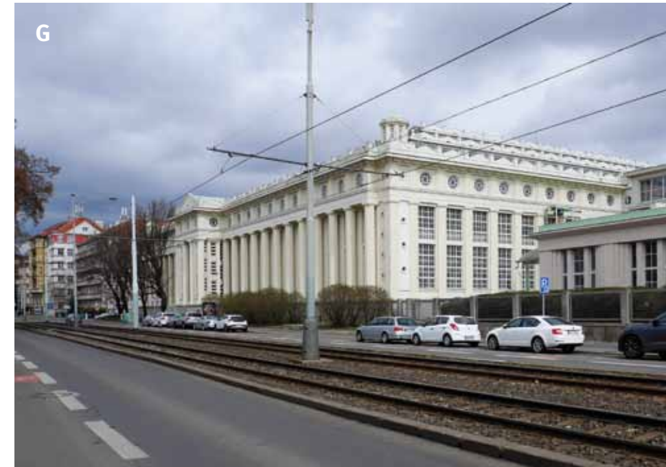
Fig. 4.233: Prague-Podolí water treatment plant: (A) original filtration hall in the 1930s; (B), (C) and (D) filtration hall; (E) and (F) clarifier hall; (G) original filtration hall. Photograph (A) – (F) by the PVK archive and Jaroslav Beneš, 2018; (G) by Michaela Ryšková, 2021.
