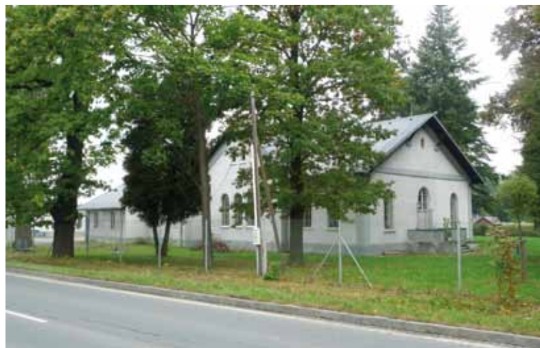
Fig. 4.194: Opava – waterworks complex in Jaselská street from 1875 with the original steam engine room building. Photograph by Alena Borovcová.
