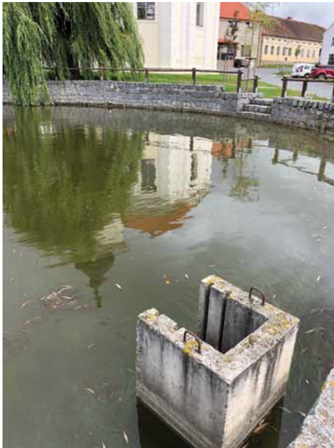
Fig. 4.62: Zbýšov – the original bottom outlet of the extinct Noový Pond with preserved relics of a pipeline pit and stilling basin. Photograph by Jindřich Frajer, 2020.
