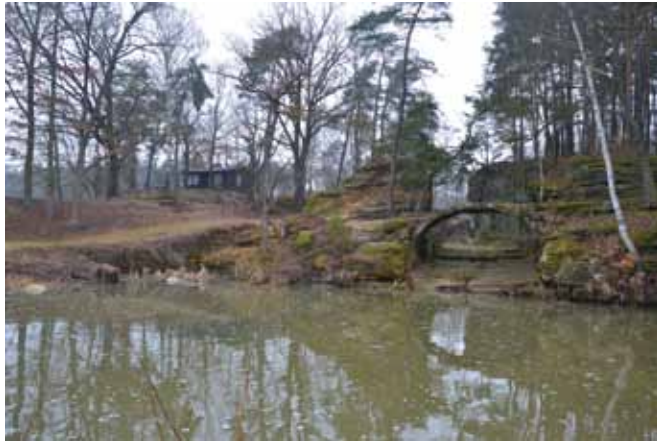
Fig. 4.66: Stvolínky, Mlýnský/Hrázský Pond – the main outlet of the pond with a bridge; to the left of it, a safety spillway. Photograph by Miroslav Kolka, 2013.
