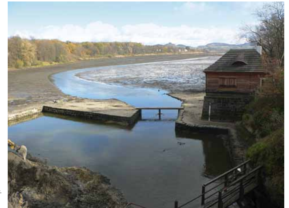
Fig. 4.70: Zahrádky, Novozámecký Pond – fishing ground with a reconstructed fishing house in front of the pond sluice gate outlet, walled by sandstone blocks. Photograph by Miroslav Kolka, 2006.
