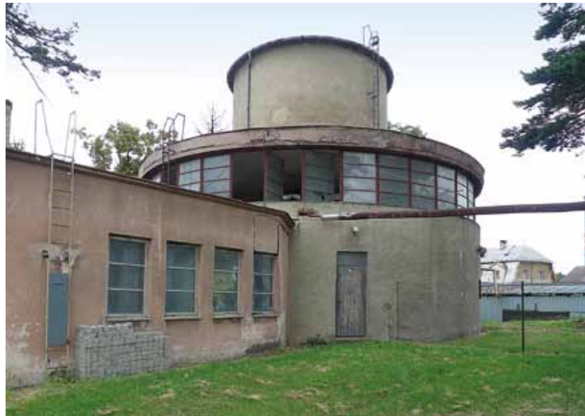
Fig. 4.223: Krnov – elevated water tank on the premises of the Karnola plant. An elevated water tank with unknown date of origin and authorship intended for non-potable water for the Karnola textile plant. A low-height water structure with a cylindrical tank carried by steel shanks and an architecturally designed casing, composed of two cylinders of different scales and broken by two horizontal ribbon windows. It was demolished in 2020. Photograph by Michaela Ryšková, 2013.
