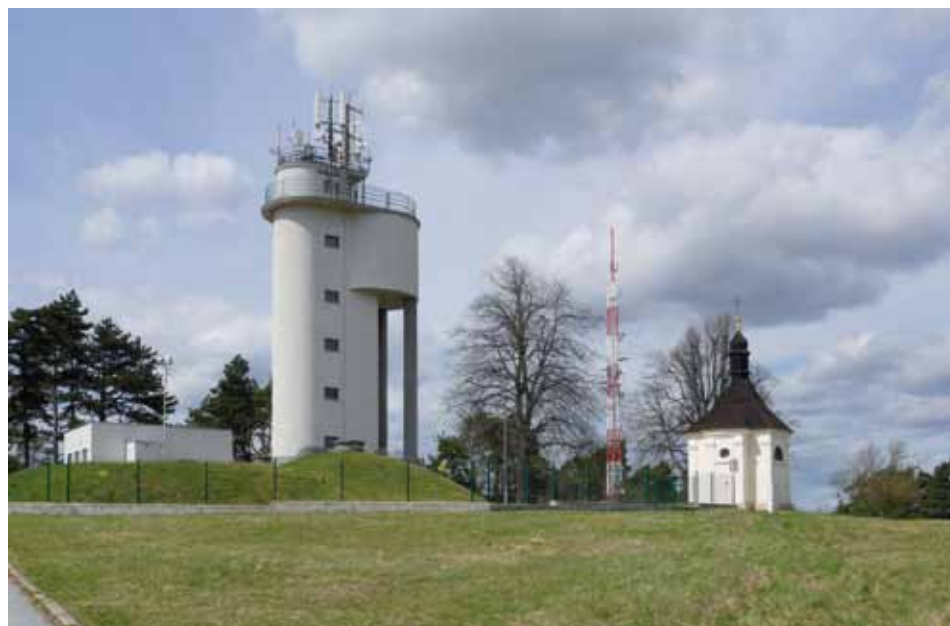
Fig. 5.24: Třebíč – “Kostelíček” elevated water tank on the Strážná hora mountain. Photograph by Michaela Ryšková, 2021.
