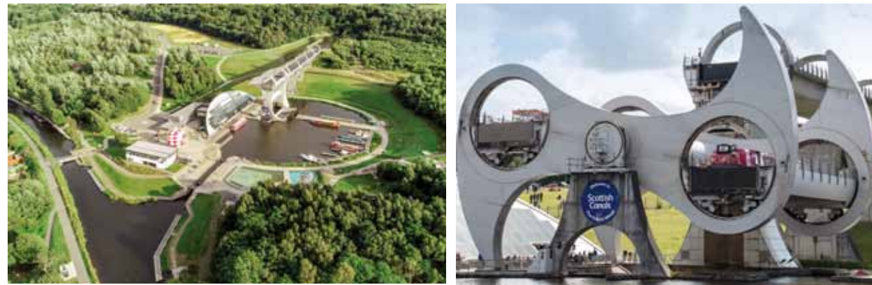
Fig. 4.82: Falkirk (Great Britain, Scotland), a rotating boat lift. Photograph by Shutterstock, 2015.
