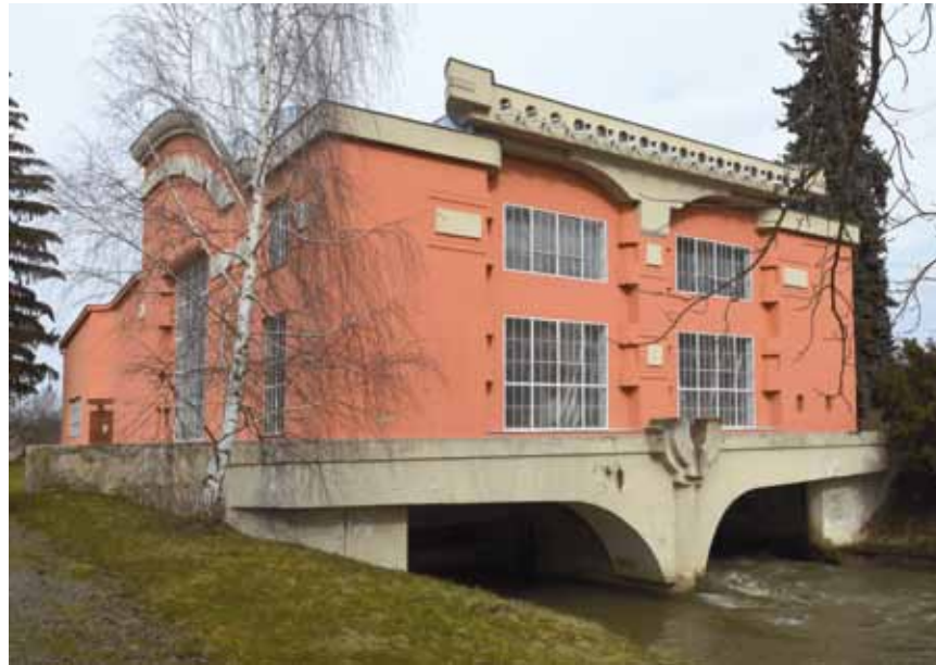
Fig. 3.15: Třeština, Háj hydroelectric power plant (1922–1923) designed by architects Bohuslav Fuchs and Josef Štěpánek. Its function is expressed in its architectural language: the architectural elements depict the energy contained in the water and its transformation and concentration. Photograph by Viktor Mácha, 2019.
