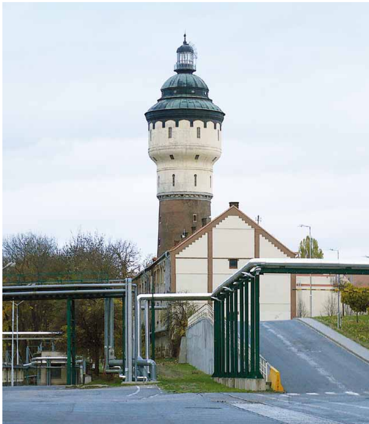
Fig. 4.196: Plzeň – elevated water tank in the premises of the Prazdroj brewery from 1905–1907 was part of the aqueduct of the City's Brewery. The implementation project was prepared by Ing. Spálek and by the builder Hucl. Two iron tanks were placed above each other, one for the spring and the other for the river water. The waterworks system consisted, besides the elevated water tank from a power plant powering the river pumping station, of coarse filter, iron removal station and sand washing machine structures and the waterworks buildings by the well Na Roudné. Photograph by Alena Borovcová, 2020.
