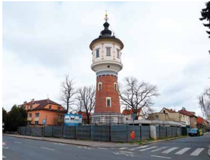
Fig. 5.22: Prague-Libeň – Na Mazance elevated water tank – after reconstruction and conversion into a flat. Photograph by Michaela Ryšková, 2022.
