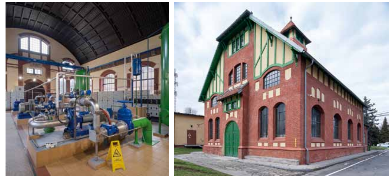
Fig. 5.2: Ostrava – water treatment plant, machine room. Photograph by Viktor Mácha, 2019.
