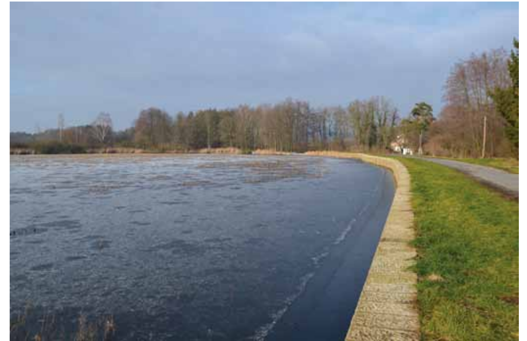
Fig. 4.51: Holany, Holanský Pond – a concave shape of a dam with a restored upstream wall from sandstone blocks. Photograph by Miroslav Kolka, 2018.
