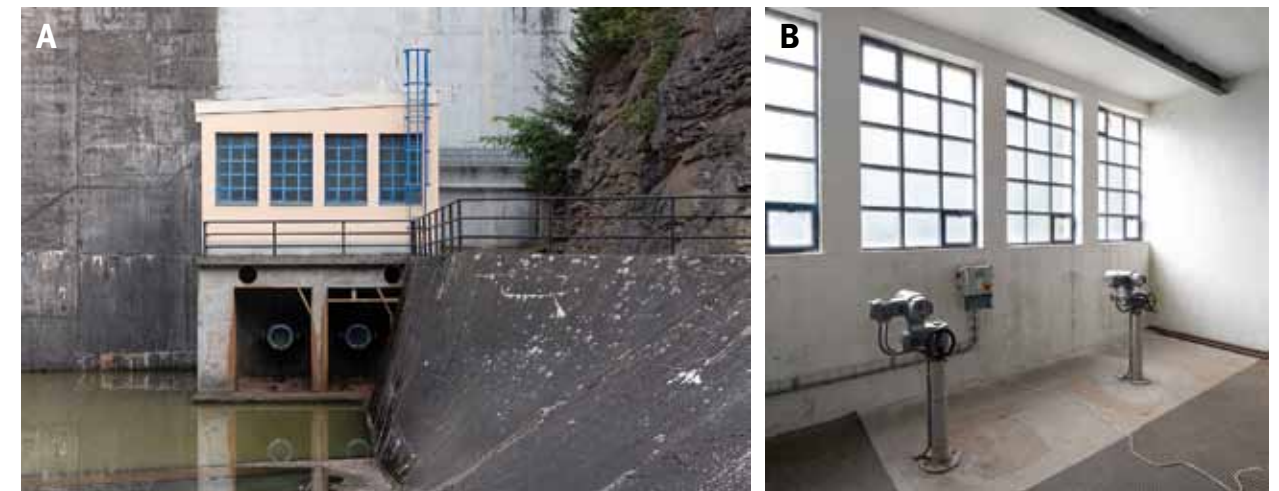
Fig. 4.24: The Vrchlice dam (1966–1970) – arch dam: (A) operational Howell Bunger valve of bottom outlets; (B) control equipment of Howell Bunger valves. Photograph by Viktor Mácha, 2020.
