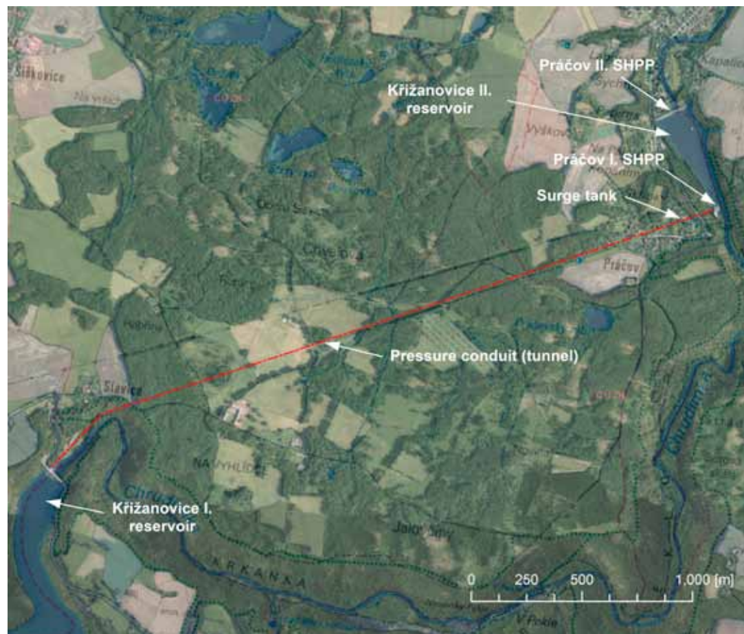
Fig. 4.137: Dam-derivation situation of the Práčov I SHPP and the Práčov II SHPP situated below the dam. Diagram created on the basis of the ČÚZK data, 2021.
