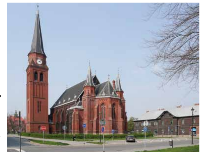
Fig. 4.221: Ostrava-Vitkovice – a unique elevated water tank in the tower of St. Paul's Church in Ostrava-Vitkovice. The town of Nové Vitkovice, founded by the Vitkovice Ironworks as a base for growing production plants, started to be built in the 1870s. St. Paul's Church with a detached tower became a significant dominant feature of its square, in addition to the town hall. The tower was built before the temple nave itself in 1882 and in its upper part there were, apart from a belfry and fire observation tower, also two tanks, each with a volume of 50 m 3 . They were part of the water supply system to which residential units and other buildings of the newly built town were connected (Matěj et al., 1992). Photograph by Michaela Ryšková, 2019.
