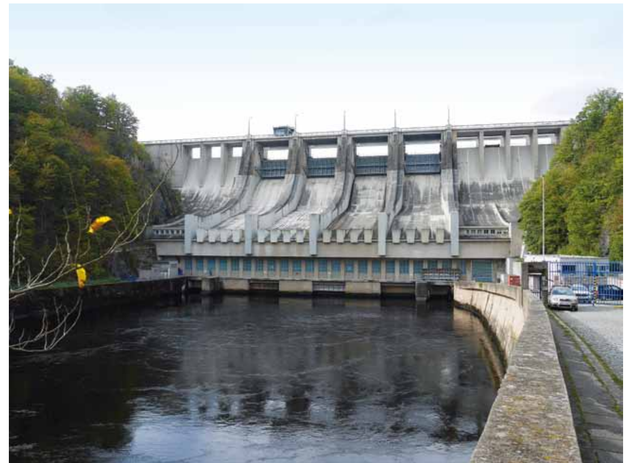
Fig. 4.41: The Slapy dam (1949–1957) – concrete gravity dam, crown safety spillway with four sections controlled by a lifting gate. Photograph by Viktor Mácha, 2021.
