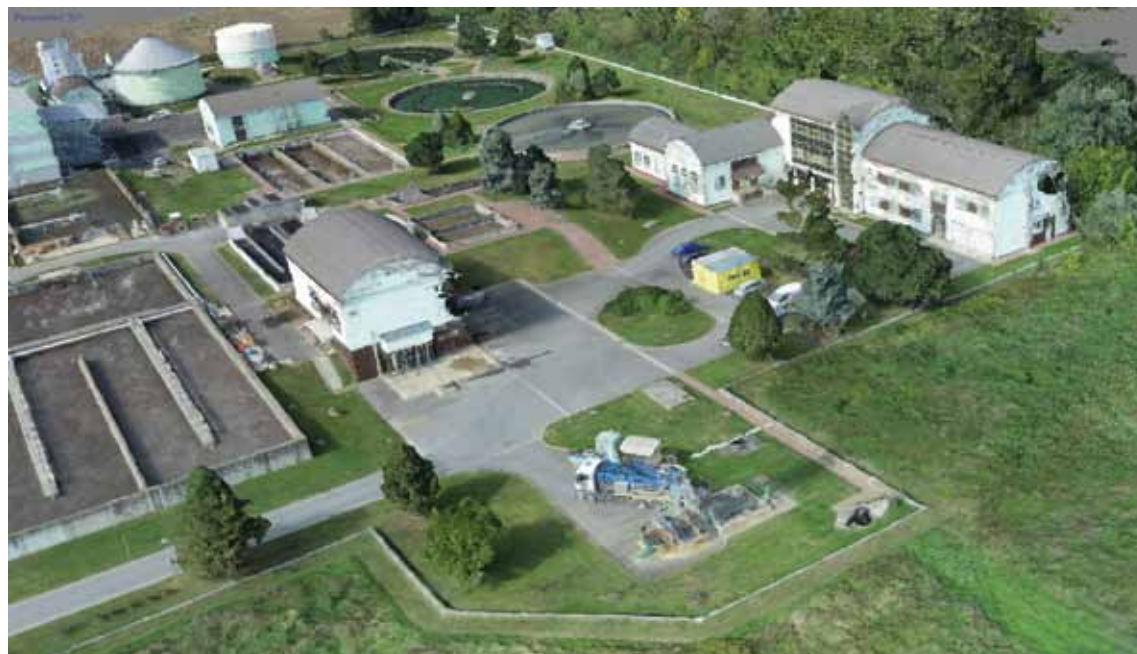
Fig. 4.273: A cutout of the final 3D model of the WWTP. Radek Bachan, 2021.
