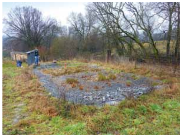
Fig. 4.258: Domestic reed-bed treatment plant. Photograph by Jaroslav Sova, 2021.
