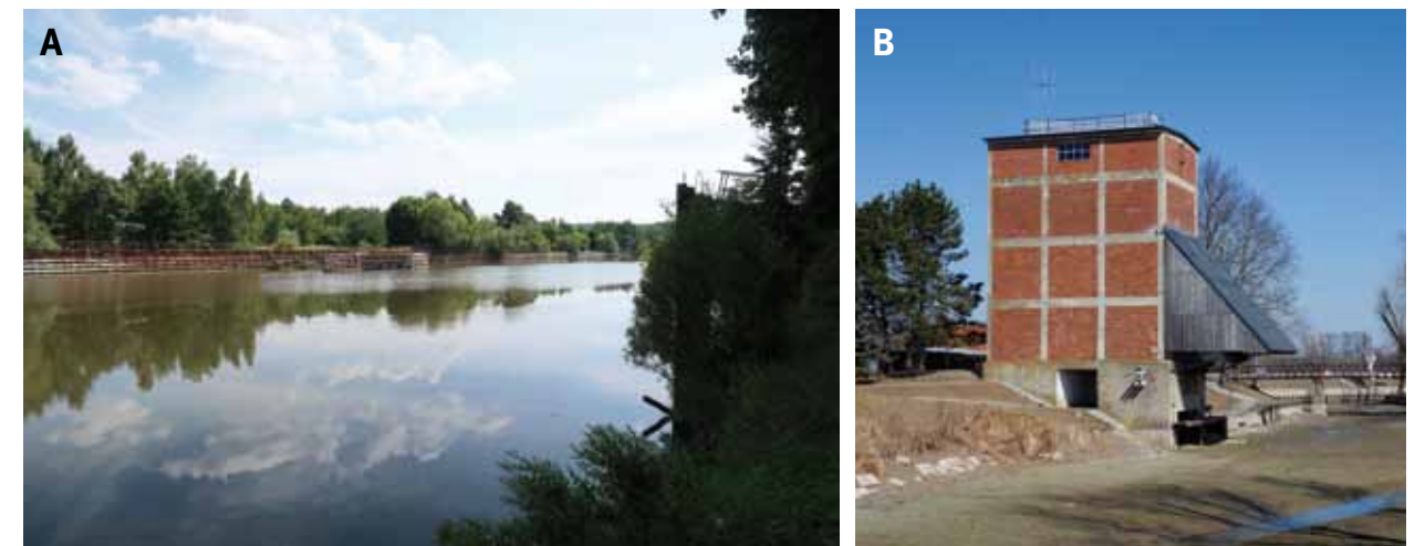
Fig. 4.76: (A) the port of Chvaletice after coal stopped being transported by water; (B) a coal tippler on the Baťa Canal near Sudoměřice. Photograph (A) by Miriam Dzuráková, 2021; (B) by Michaela Ryšková, 2022.
