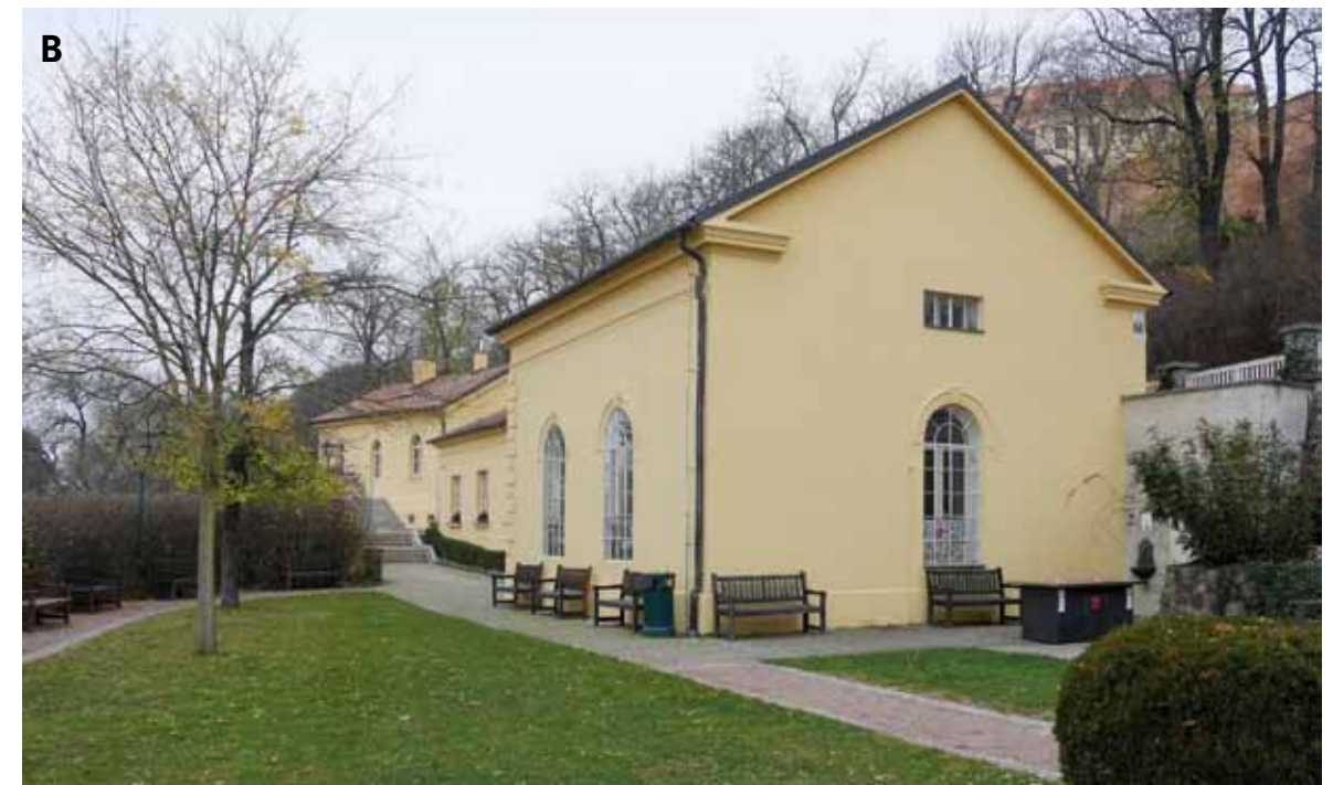
Fig. 3.10: Former pumping stations: (A) Opava, (B) Brno. The appearance of this former steam-powered pumping station is characteristic of this type of building. It was a single-floor structure with a gable roof and windows incorporating semicircular upper sections. Photograph (A) by Alena Boroucová and (B) by Michaela Ryšková, 2021.
