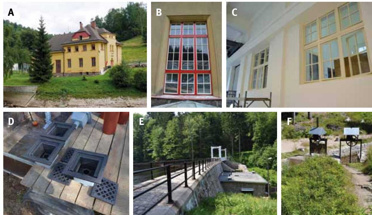
Fig. 5.8: Rudolfov – reconstruction of the hydraulic structure and power plant: (A) facade after renovation; (B) new simple exterior glass panels in the machine room with the facade before renovation; (C) interior glass and door panels were preserved in the original form and overhauled; (D) renovation of a non-functional system of a surge chamber dam with refurbishment and graphite painting of dewatering elements; (E) dam after the painting of railings with the SHPP II building had been completed (on the right); (F) renovation of all collecting structures on the conduit. Photograph by Petr Freiwilg, 2020.
