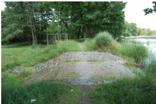
Fig. 4.68: Rašsko, Vavroušek Pond – safety spillway. Photograph by Miroslav Kolka, 2012.
