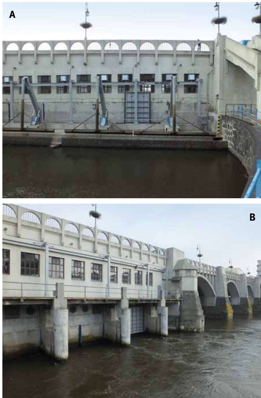
Fig. 4.141: Kolín SHPP: (A) inlet structure; (B) outlet structure. Photograph by Brno University of Technology, Faculty of Civil Engineering, 2015.
