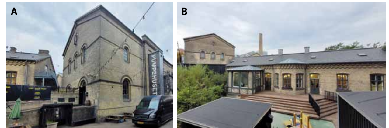
Fig. 5.19: Copenhagen (Denmark) – pumping station ( Pumpehuset ): (A) former machine room building, today a venue for concerts; (B) water inspector's former residence, today kindergarten premises. Photograph by Viera Dedíková, 2021.
