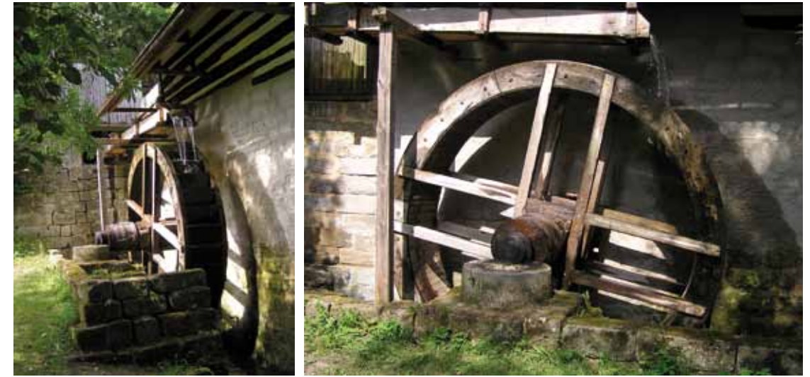
Fig. 4.165: Střehom (Mladá Boleslav District) – overshot bucket water wheel. Photograph by Radim Urbánek, 2006.
