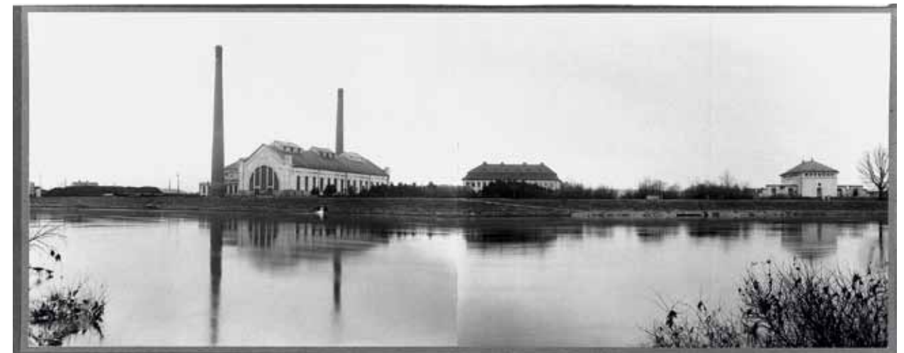
Fig. 4.202: Káraný, Káraný waterworks – waterworks at the confluence of the Labe and Jizera, built from 1896 to 1912, launched in 1913, officially launched on 1 January 1914. It was founded to collect underground water, which appeared due to leakage of river water to suitable, in this case gravel-sand, subsoil. Naturally filtered water is captured by underground sucking wells. In the 1960s the process was complemented with artificial infiltration which was connected with direct pumping of raw water from the river through a system of outdoor sand filters. A secondary water source is a system of artesian wells. Originally it was powered by steam engines but in the 1930s it was upgraded to electric power. The waterworks is still fully operational. From the outset it concerned a local group water supply network because the original consumer base was Prague and its suburbs, and from the second half of the 20th century a range of neighbouring villages located along the main conduit were connected to the system. Photograph: the PVK archive, fonds Fotoarchiv PVK, box N 21, sign. C 083a.
