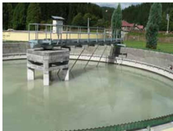
Fig.4.244: Radial settling tank. Photograph from the TGM WRI archive.
