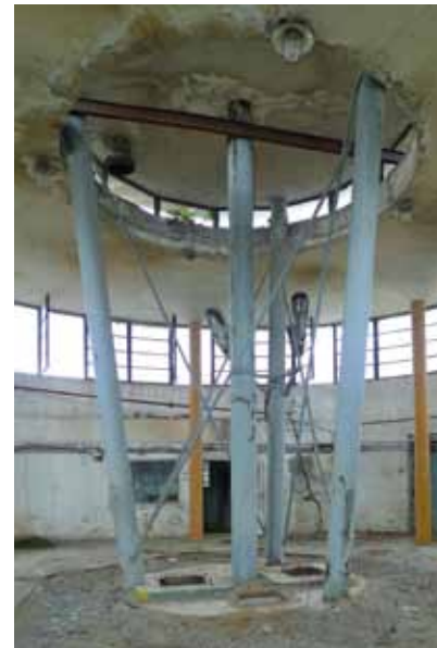
Fig. 4.223: Krnov – elevated water tank on the premises of the Karnola plant. An elevated water tank with unknown date of origin and authorship intended for non-potable water for the Karnola textile plant. A low-height water structure with a cylindrical tank carried by steel shanks and an architecturally designed casing, composed of two cylinders of different scales and broken by two horizontal ribbon windows. It was demolished in 2020. Photograph by Michaela Ryšková, 2013.
