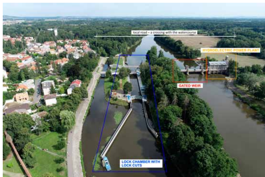
Fig. 4.120: The Poděbrady navigation lock – functional complex elements. Photograph by Radek Bachan, 2021.
