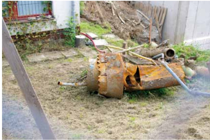
Fig. 5.28: The fitting of the secondary settling tank damaged during the renovation of the water treatment plant. Photograph by Miloš Rozkošný, 2021.
