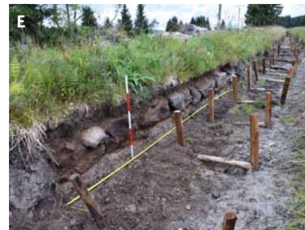
Fig. 5.13: Blatná Water Ditch: (A) forest part of the watercourse, state before reconstruction; (B) historic boundary mark on the border of the watercourse plot; (C) trough after the removal of worn out timbering; (D) ramming of the trough new timbering; (E) Blatná Water Ditch near Kozí Sejfy just above Horní Blatná, example of neatened bank armouring uncovered by the construction; (F) water ditch near Kozí Sejfy above Horní Blatná, example of sedimentation profile (the oldest one?) of the river bed uncovered by the construction. Layers of carbons and the absence of clay insulation are evident at the bed sitting on yellow coarse stone material. Layers of alluvial sand are also well distinguishable. Photograph (A) – (D) by Jakub Chaloupka, (E) and (F) by Ondřej Malina, 2021.
