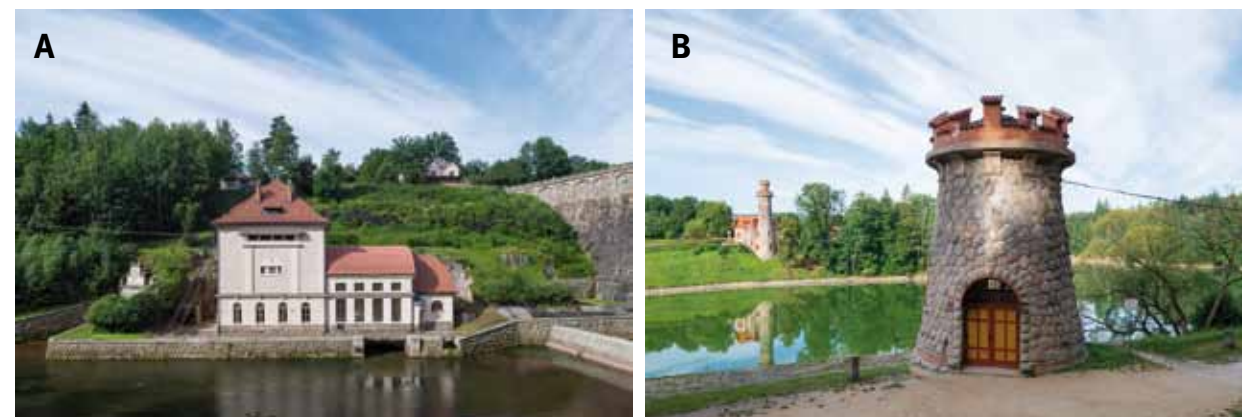
Fig. 4.39: The Les Království dam (1910–1919): (A) hydroelectric power plant building; (B) valve tower to control bottom outlets in the left by-pass tunnel; in the background, the dam keeper's house. Photograph by Viktor Mácha, 2020.
