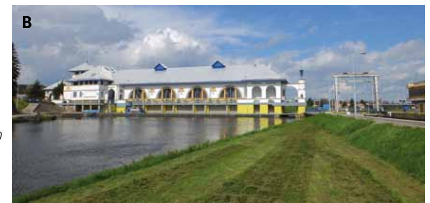
Fig. 4.125: Miřejovice SHPP on a short headrace: (A) diagram; (B) a view of the inlet part. Diagram (A) created on the basis of the ČÚZK data, 2021; photograph by Brno University of Technology, Faculty of Civil Engineering, 2014.
