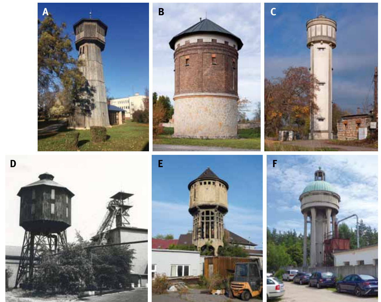
Fig. 4.217: Examples of supporting structures of water tanks: (A) Palárikovo (Slovakia), wooden elevated water tank, probably the only surviving one in Europe, after conversion; (B) Kovanec, elevated water tank with masonry wall supporting structure from stone and bricks, built in the historicist morphology according to Karel Kress's design in 1909; (C) Horní Bukovina, elevated water tank with reinforced concrete supporting structure built in 1935 according to Ing. Fanta's design; (D) Ostrava, Hubert mine, extinct elevated water tank with steel supporting skeleton (framed) structure and wooden cladding of the tank in the picture from the end of the 1960s; (E) Duchcov, elevated water tank with a skeleton reinforced concrete supporting structure built between 1908 and 1912 for the Engels glassworks; (F) Lázně Bohdaneč, an elevated water tank supported by a reinforced concrete combined structure, built according to Josef Gočár's design in 1911, in the middle shank of the structure there is a staircase. Photograph (A), (E) and (F) by Michaela Ryšková, 2021, 2020, 2016; (B) and (C) by Viktor Mácha, 2018; (D) from the MCPD reprophotography archive.
