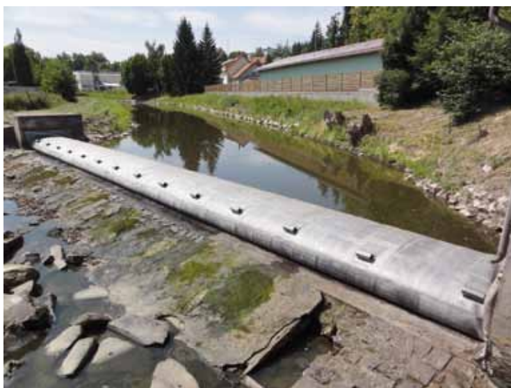
Fig. 4.112: Jihlava, an inflatable weir on the Jihlava River. Photograph from the Brno University of Technology archive, 2013.
