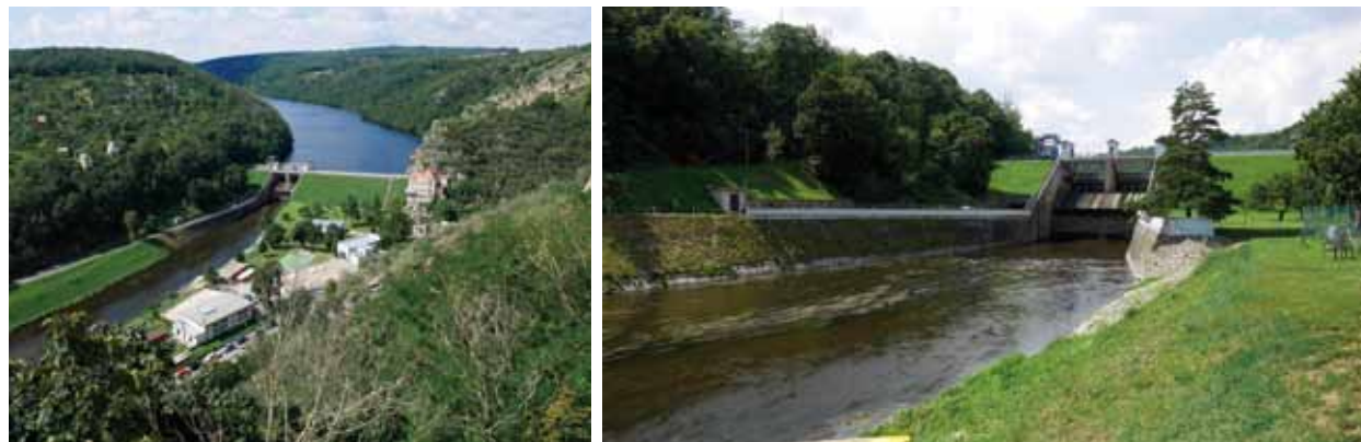
Fig. 4.17: The Znojmo dam (1962–1965) – composite dam. Photograph by Michaela Ryšková, 2020.
