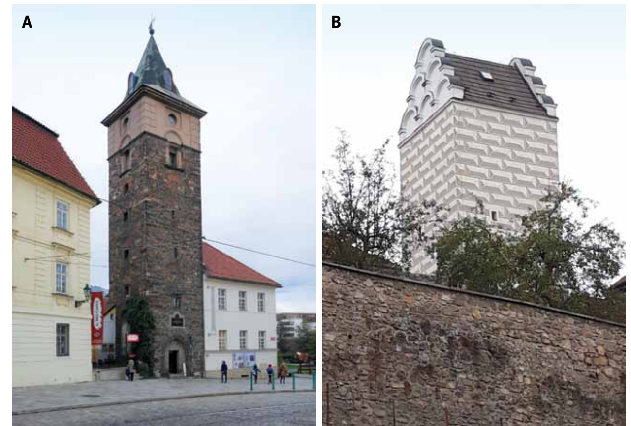
Fig. 3.9: Water towers: (A) Plzeň, late Gothic water masonry water tower, first documented in 1532. The Classicist pumping station (right) was built using stone from the city's demolished Prague Gate. The Gothic-inspired shape of the roof evidently dates from 1845, when the tower was raised as part of a reconstruction project carried out by the contractor Kristian Lexa. In 1843 the upper level of the tower contained a copper tank with a volume of 2.7 m 3 . The pumping station was equipped with a metal-plated water wheel and a three-cylinder pump; it drew water from the river. The entrance portal, added during the 19th century, was originally from a house in the city (Hlušíčková 2003). (B) Tábor, the Renaissance tower, with its sgraffito inscriptions and arched gables, was built after a fire in 1559. The town was supplied with water from the Jordán valley reservoir (1492); below the dam there was a pumping station with a wooden pump driven by a water wheel, which pumped water into a tower that supplied the municipal fountains (Vávra 1913). Today the building houses a gallery. Photograph (A) by Alena Boročková, 2020 and (B) by Eva Dvořáková.
