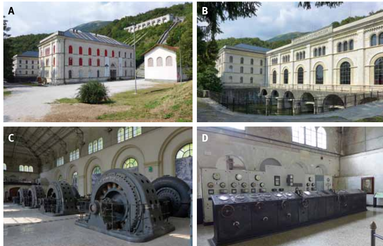
Fig. 5.16: Malnisio di Montereale Valcellina (Italy): Antonio Pitter hydroelectric power plant. Photograph by Michaela Ryšková, 2016.
