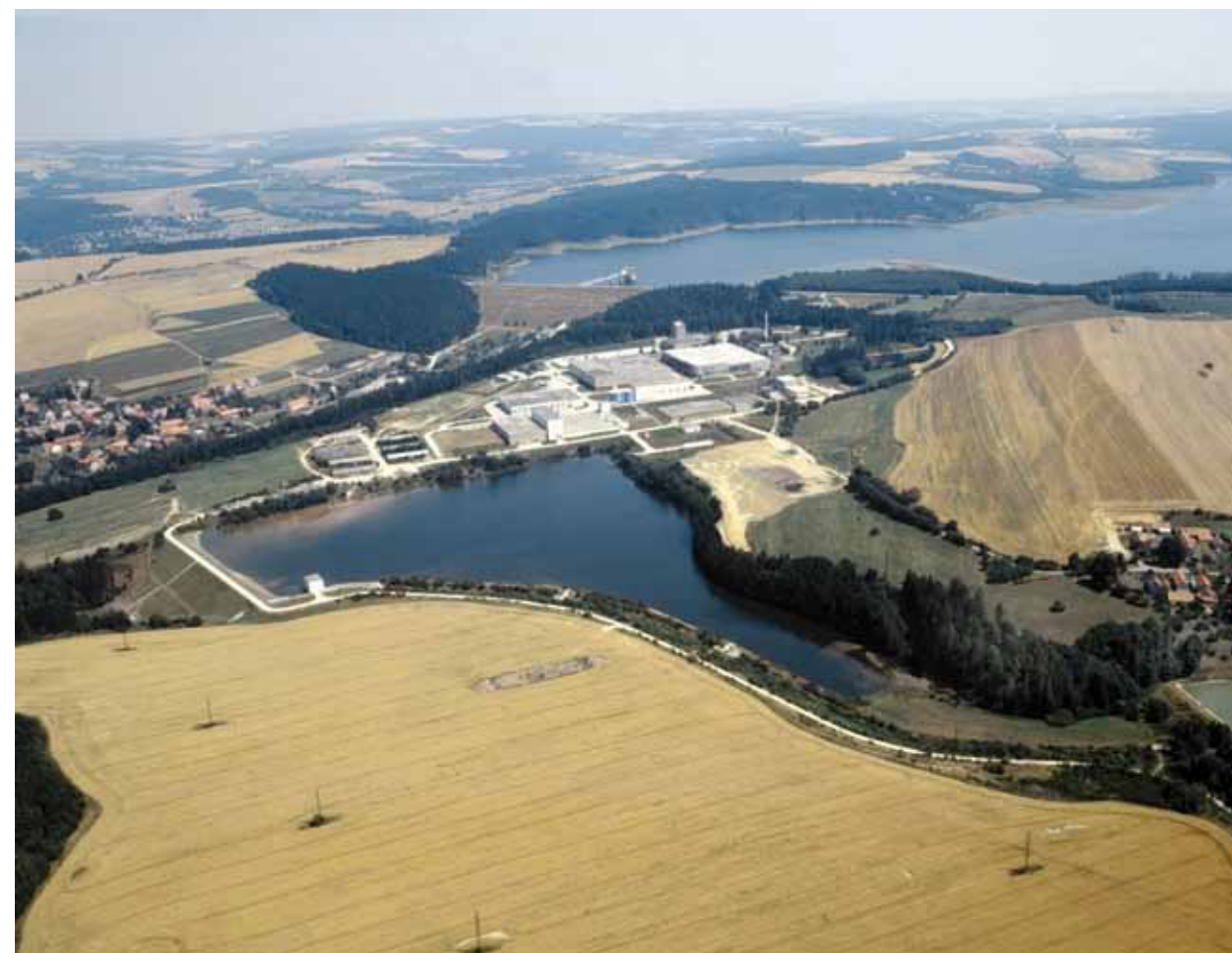
Fig. 4.229: Švihov – aerial view of the Želivka water treatment plant. Photograph from PVK archive, fonds Fotoarchív PVK, box N 17, sign. B 180/00.
