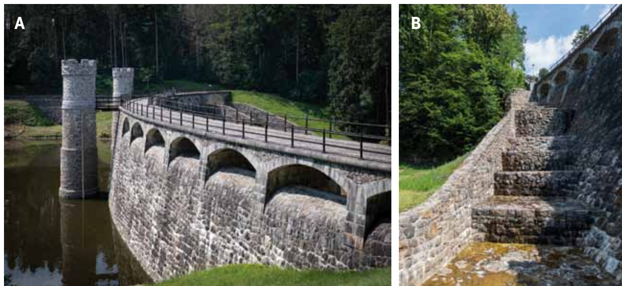
Fig. 4.12: The Pařížov dam (1909–1913): (A) the view on the crown safety spillway from the upstream side; (B) the view from the downstream side on the crown spillway cascade. Photograph by Viktor Mácha, 2020.
