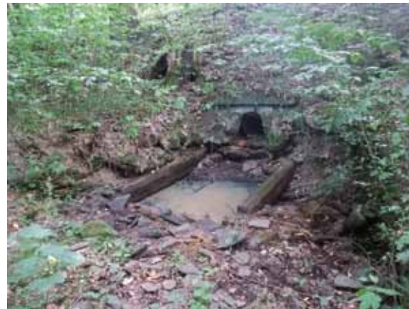
Fig. 4.62: Zbýšov – the original bottom outlet of the extinct Noový Pond with preserved relics of a pipeline pit and stilling basin. Photograph by Jindřich Frajer, 2020.
