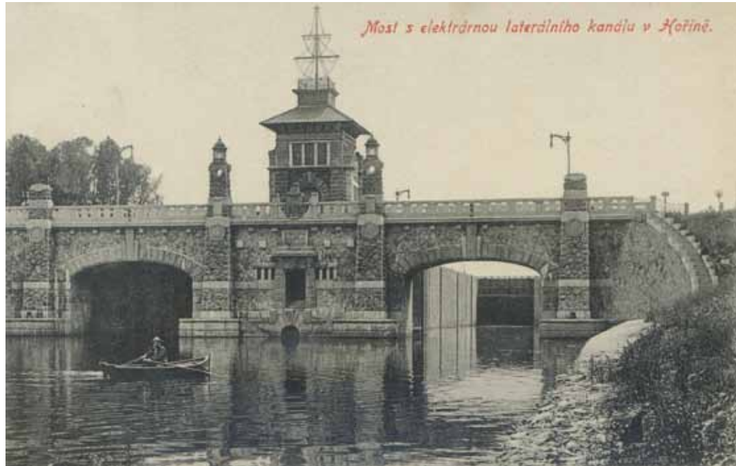
Fig. 3.11: Hořín, lock chambers, bridge and power plant on the Vraňany–Hořín lateral canal. Historical postcard, collection of Michaela Ryšková.
