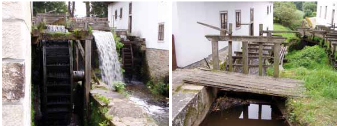
Fig. 4.89: Ratibořice, wooden elements of the mill race at Granny's valley. Photograph by Milena Forejtníková, 2010.
