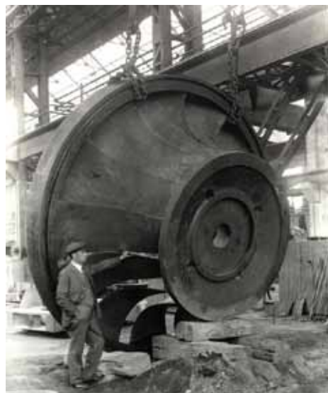
Fig. 4.178: Production of the Francis turbine runner for the Miřejovice SHPP (taken from: ČKD Blansko company materials).
