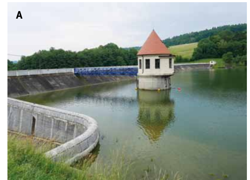
Fig. 4.208: Free-standing multipurpose structures for the withdrawal of water from reservoirs: (A) Fryšták reservoir, free-standing multipurpose structure of outlets and water-supply intakes with a machine room for the control of outlet gates in the upper part. The withdrawal of water is ensured by two pipelines at two levels. Part of the hydraulic structure is also a water treatment plant situated under the dam of the reservoir. (B) Švihov hydraulic structure, source of raw water for the Želivka water treatment plant. Free-standing multipurpose intake structure of the dam. The withdrawal of water is ensured by two intake buttresses with the possibility of five-level intakes reaching up to the bottom of the reservoir ended by an emergency overflow at the crest. Water is led into a pumping station at the heel of the dam and then into the water treatment plant (Parkán and Pěkný, 2012). Photograph (A) by Michaela Ryšková, 2020; (B) from PVK archive.
