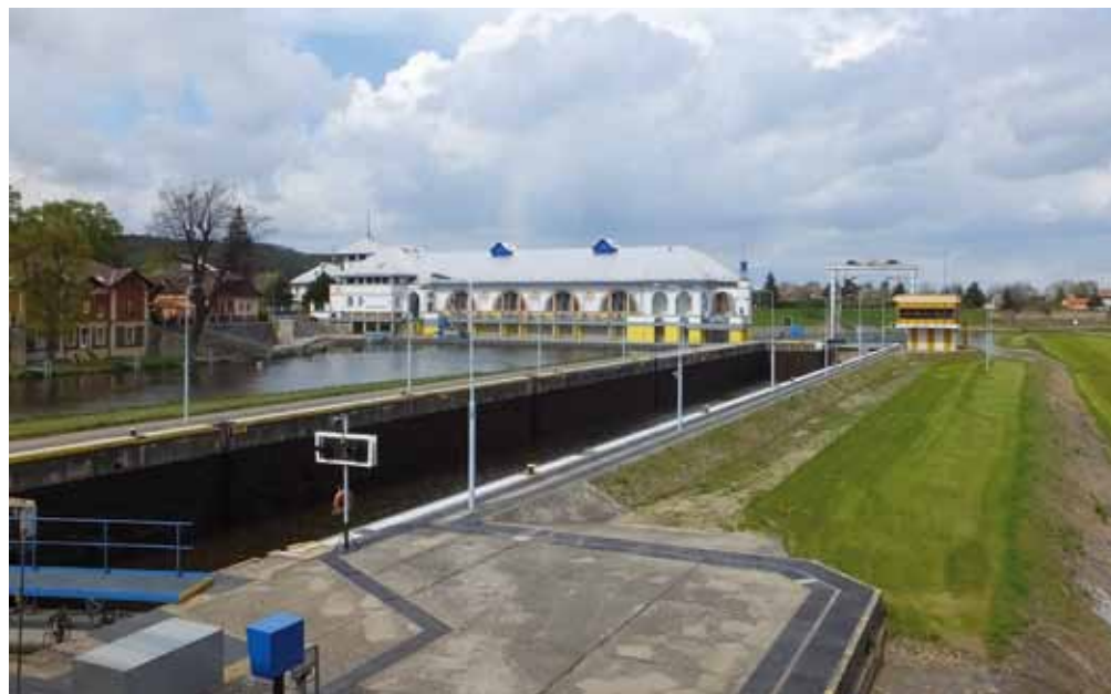
Fig. 4.187: Miřejovice SHPP with a lock chamber. Photograph by Aleš Dráb, 2014.
