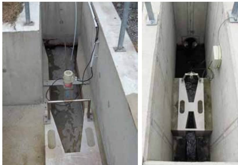
Fig. 4.255: The Purshall flume, an ultrasound sensor for the measurement of water flow. Photograph from the TGM WRI archive.
