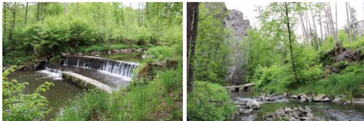
Fig. 5.26: Křemžský Brook – On the left, a view of the lowest situated navigation lock. On the right, a view of one of the contemporary bridges – prefabricated concrete. Photograph by J. Hansová, 2021.
