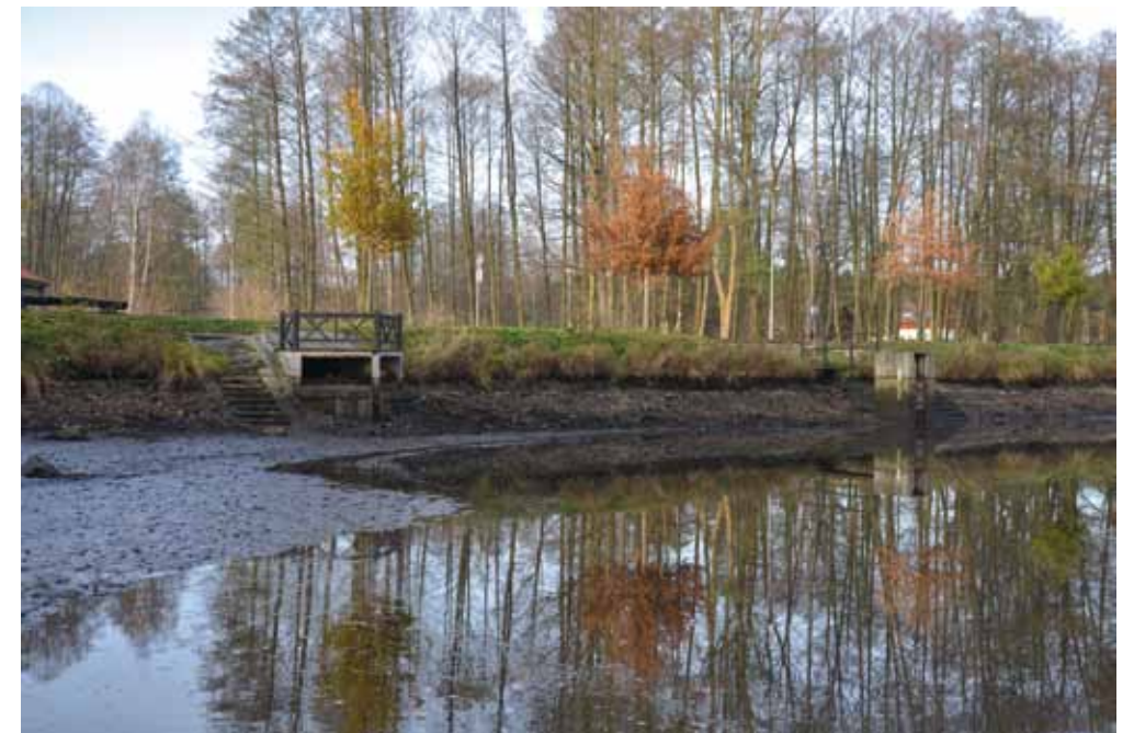
Fig. 4.52: Hradčany, Hradčanský Pond – a straight dam with a main outlet (on the right) and a discharge to the race to the extinct mill (on the left); state after the pond drawdown. Photograph by Miroslav Kolka, 2017.
