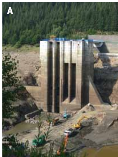
Fig. 4.146: Dlouhé Stráně PSHPP, lower reservoir – tower inlet structure (multipurpose – it also contains bottom outlets and safety spillways): (A) state during the reservoir drawdown; (B) section: 1 – machine room of safety spillways radial gates, 2 – bridge, 3 – backfill, 4 – rack or temporary flashboards (stop logs), 5 – slide gate valve, 6 – gunite, 7 – sealing element of expansion joints. Photograph (A) by Brno University of Technology, Faculty of Civil Engineering; diagram (B) by Radka Račoch and Michaela Mrosová, 2021 (modified according to Hynková, 1984).
