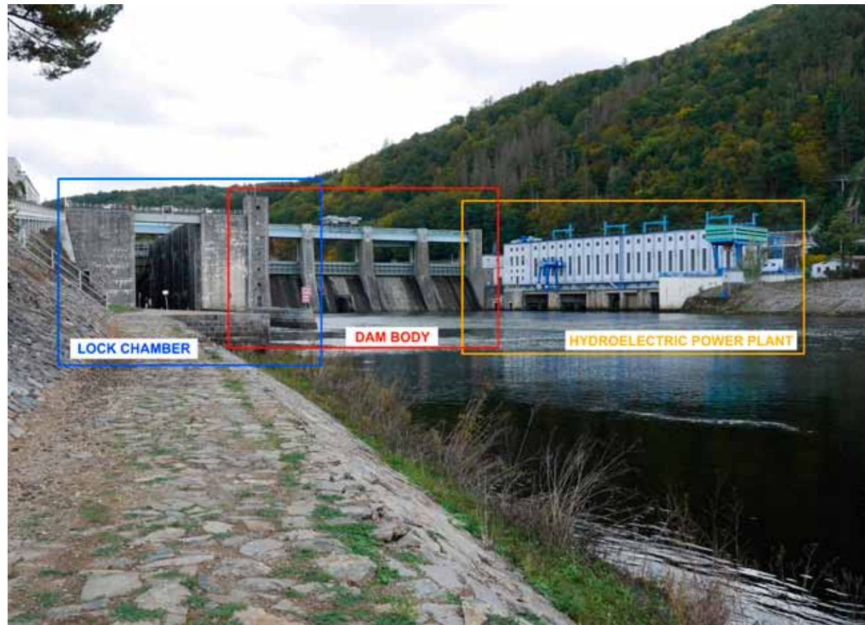
Fig. 4.35: The Štěchovice HS (1937–1945) – concrete gravity dam. Example of a functional complex – dam + lock chamber + hydroelectric power plant. Photograph by Michaela Ryšková, 2020.
