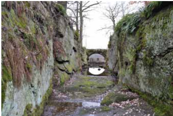
Fig. 4.67: Stvolínky, Dolanský Pond – a rock gully of the safety spillway; in the background a bridge in the dam route. Photograph by Miroslav Kolka, 2016.
