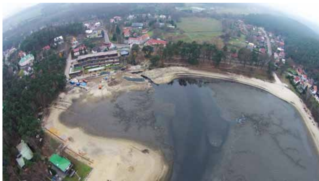
Fig. 4.50: Doksý – Staré Splavy, Mácha Lake – In the left part of the picture, a straight dam of a pond which consists of an outcrop of a sandstone bedrock with a basalt vein, in the middle part there is an outlet gully; state during the reconstruction of the outlet structure and the pond drawdown. Photograph by A. Kopecký, 2014.
