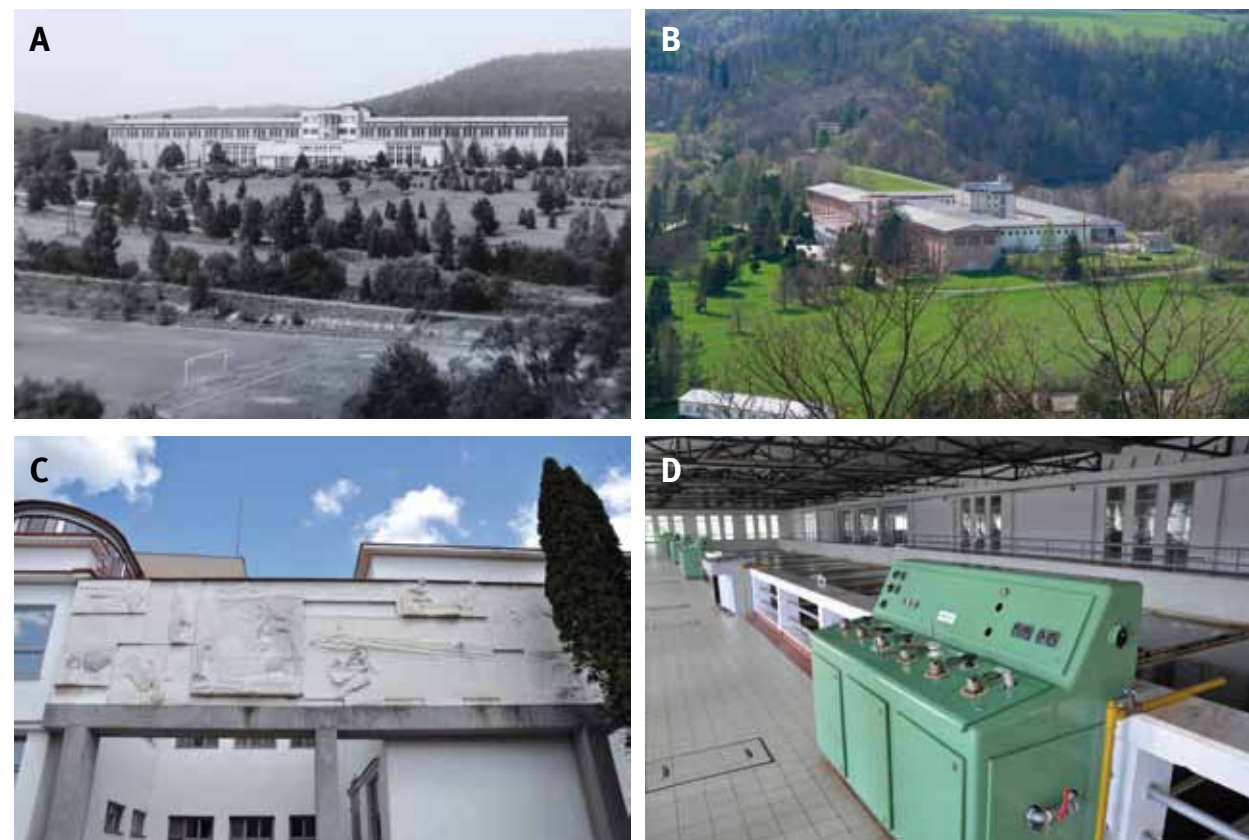
Fig. 5.3: Vítkov-Podhradí – water treatment plant: (A) original appearance (taken from: ČVVS, 1972); (B) current appearance; (C) part of Vincent Makovský's relief; (D) control panel. Photograph by Miriam Dzuráková, 2019.
