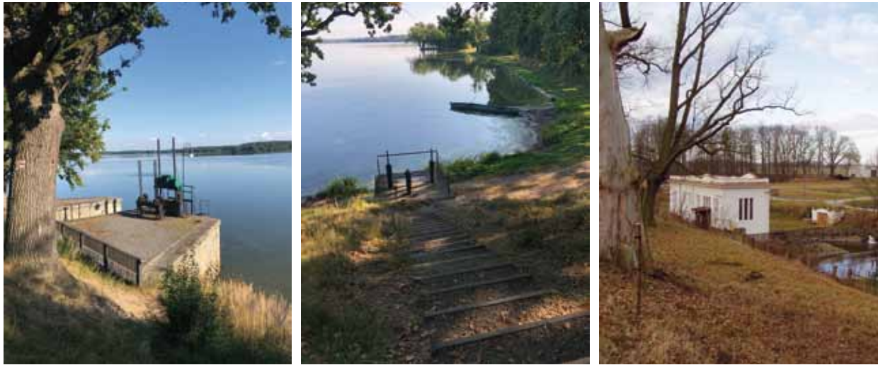
Fig. 4.72: Rožmberk Pond and outlet structures, small hydroelectric power plant built at Rožmberk Pond in 1922 and historical wooden pipeline from the pond dam. Photograph by Eva Dvořáková, 2006.
