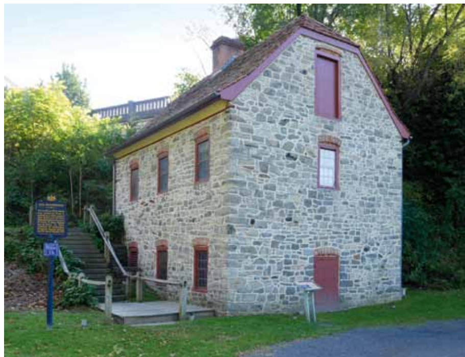
Fig. 3.23: Bethlehem (USA), pumping station. America adopted European Early Modern-era systems of water supply (16th–17th centuries) based on the principle of remote gravitational supply, using pumps driven by water wheels. The oldest water pumping station in the USA was built in 1754 for the town of Bethlehem, established by immigrants from the Moravian community. The water was pumped from a source to a water tower, from where it flowed gravitationally into five cisterns and tanks. The building in the photograph functioned as a pumping station until 1832. (Douet, 2018). Photograph by Michaela Ryšková, 2018.
