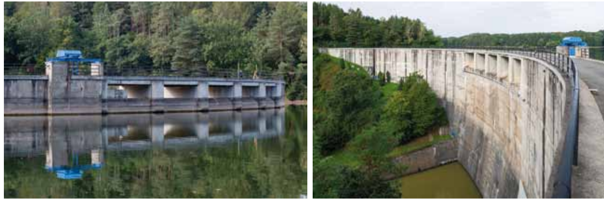
Fig. 4.21: The Vrchlice dam (1966–1970) – arch dam. Photograph by Viktor Mácha, 2020.
