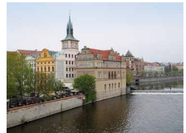
Fig. 4.191: Prague – pumping station of the Old Town Waterworks. Photograph by Michaela Ryšková, 2022.
