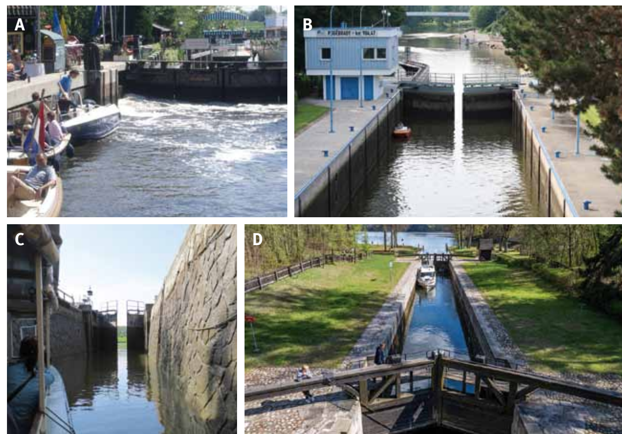
Fig. 4.79: Examples of lock chambers: (A) Netherlands, filling of a lock chamber by a gate by-pass; (B) Poděbrady, a lock chamber with steel gates filling by-pass channels openings; (C) a lock on the Bata Canal on the lower water, Cyclopean masonry; (D) Poland, a lock with wooden gates on the Augustów Canal. Photograph (A) by V. Forejtník, 2007; (B) by Miriam Dzuráková, 2021; (C) by the TGM WRI archive, 2012; (D) Milena Forejtníková's personal archive.
