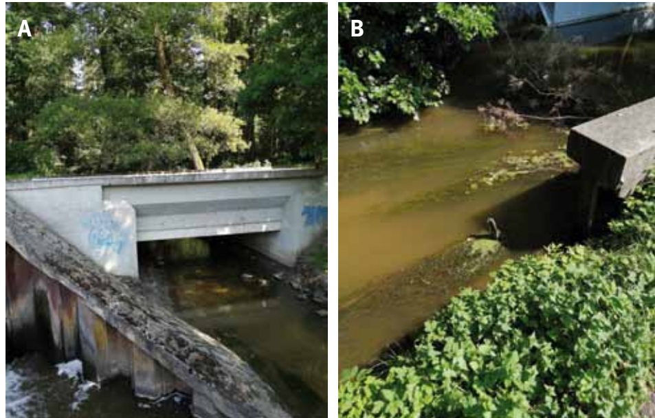
^ Fig. 4.92: The Semínský aqueduct on the Opatovice Canal: (A) state after reconstruction; (B) remains of old wooden elements. Photograph by David Honek, 2020.
