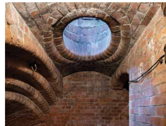
Fig. 3.24: Prague-Bubeneč, old wastewater treatment plant. This treatment plant, designed by William H. Lindley in 1894, is one of the most important European examples of a solution to the problem of wastewater – an issue faced by rapidly growing industrial cities towards the end of the 19th century. For more information see Chapter 4.6. Drainage/sewerage and water treatment. Photograph by Viktor Mácha, 2020.
