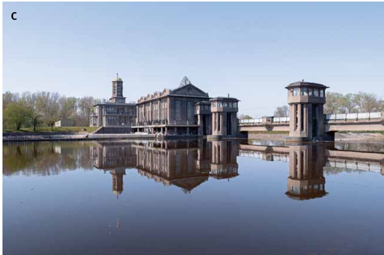
Fig. 4.121: Situation in the locality of the functional complex of the Poděbrady navigation lock: (C) weir and power plant. Photograph by Viktor Mácha, 2019.
