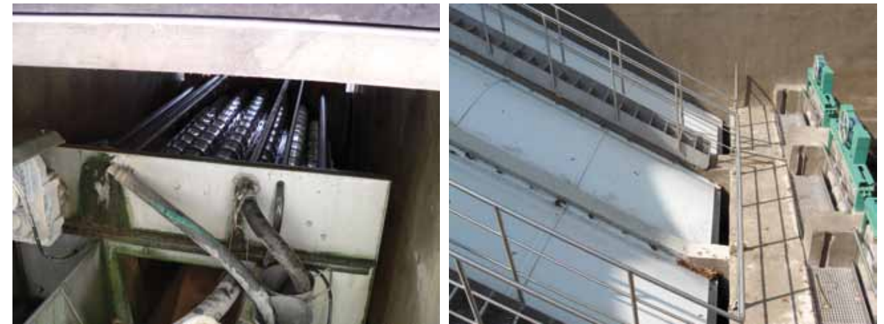
Fig. 4.242: Screw pumps. Photograph from the TGM WRI archive.
