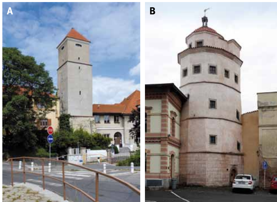
Fig. 4.188: Examples of water towers: (A) Mělník, Renaissance water tower in Pražské předměstí, probably from the 14th century, which forms a free-standing part of the town’s mediaeval fortifications; non-potable water from Pšovka Brook was pumped into its tank; it served its purpose until 1882 (Hlušíčková, 2002); (B) Nymburk, the so-called Turkish tower from the end of the 16th century was built instead of an older wooden tower. Photograph by Michaela Ryšková, 2021, 2018.
