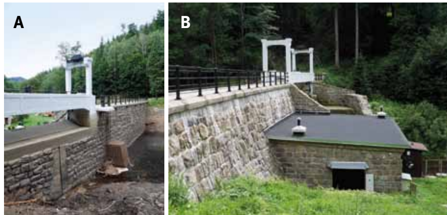
Fig. 4.132: Rudolfov II SHPP: (A) upstream slope of the dam with an inlet structure; (B) SHPP machine room. Photograph by Michaela Ryšková, 2021.
