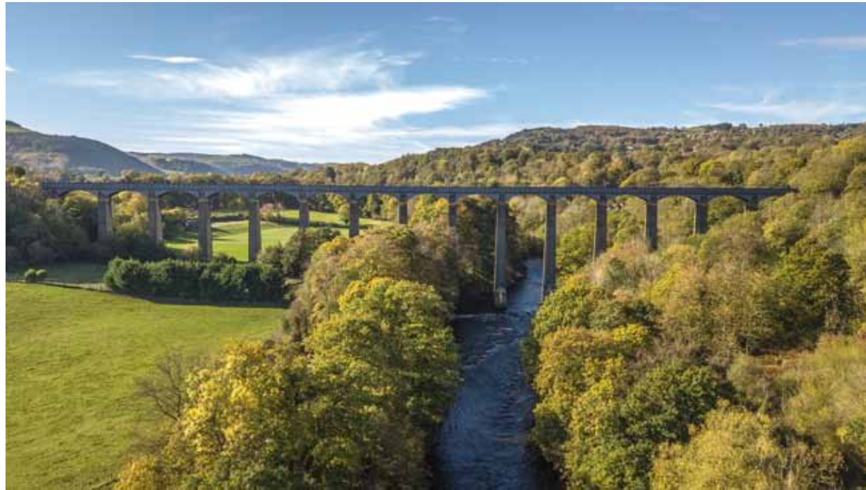
Fig. 4.85: Aqueduct Pontcysyllte (Great Britain, Wales). Photograph by Shutterstock, 2021.
