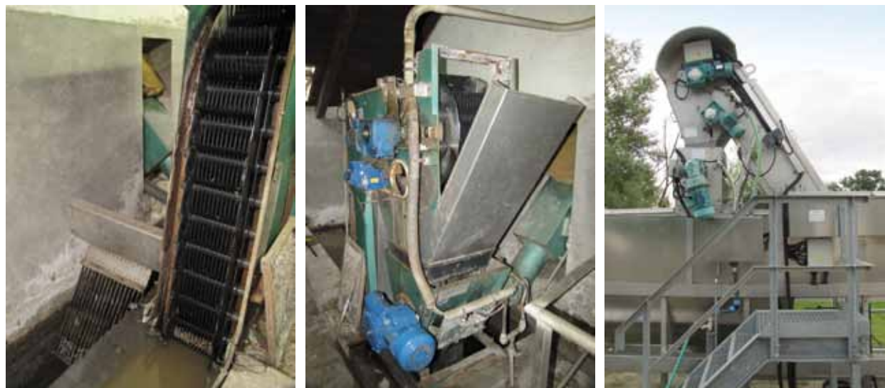
Fig. 4.239: Fine screen – machine-raked. Photograph from the TGM WRI archive.
