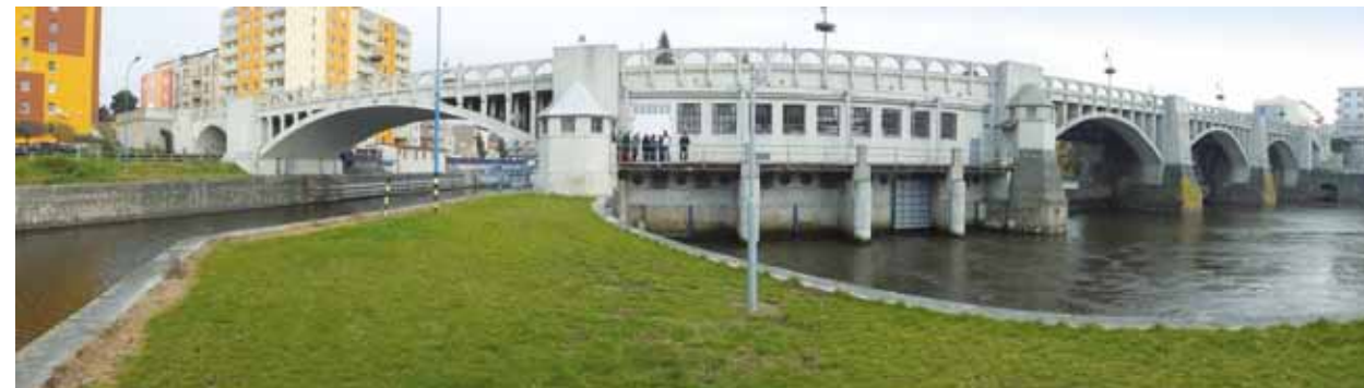
Fig. 4.131: Kolín SHPP – a view from the area downstream of the weir of the machine room and the outlet part of the small hydroelectric power plant (on the left) and three sections of the roller drum weir (on the right). Photograph by Brno University of Technology, Faculty of Civil Engineering, 2014.
