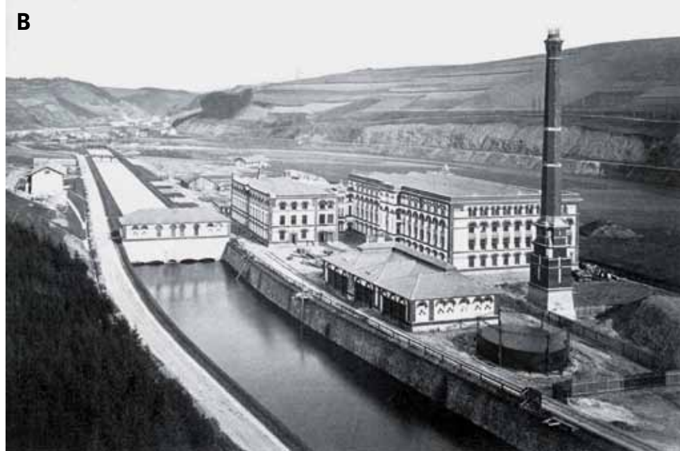
4.134: Železný Brod – current situation of the derivation channel-type small hydroelectric power plant: (A) current layout after the demolition of the original machine room and subsequent complete reconstruction with a new machine room at the end of the derivation channel; (B) historic layout with the original location of the machine room from 1897. The diagram (A) was created on the basis of the ČÚZK data, 2021; photograph (B) from the archive of the company Vodní elektrárna Železný Brod, a. s.
