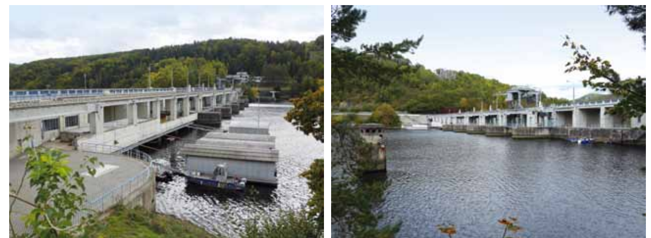
Fig. 4.42: The Slapy dam (1949–1957) – a concrete gravity dam, view of the upstream face. Photograph by Viktor Mácha, 2021 and Michaela Ryšková, 2020.
