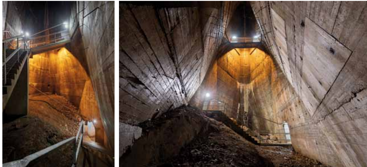
Fig. 4.19: The Fláje dam (1951–1963) – buttress dam. Photograph by Viktor Mácha, 2020.
