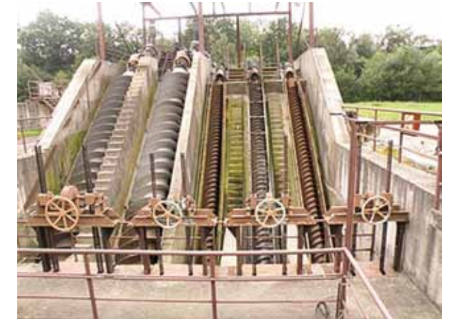
Fig. 4.242: Screw pumps. Photograph from the TGM WRI archive.
