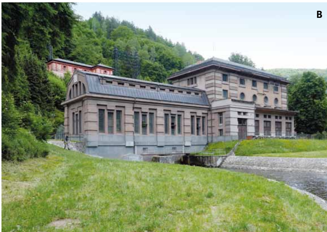
Fig. 4.152: Spálovo SHPP: (A) longitudinal section of a surge chamber, supply pressure pipeline and machine room; (B) view of the machine room and surge chamber at the end of the headrace. Diagram (A) taken from: ZČE, 2000; photograph (B) by Michaela Ryšková, 2022.
