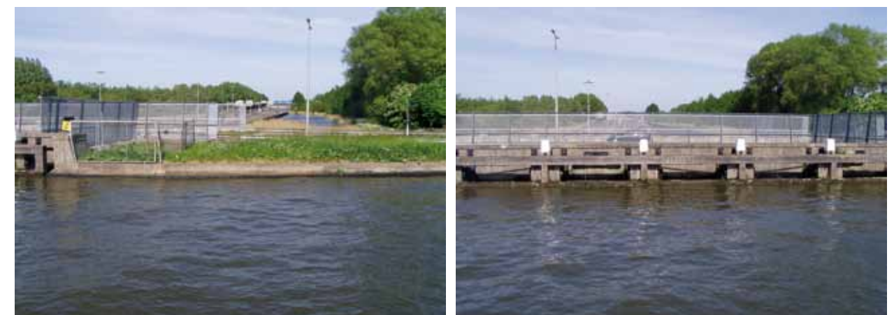
Fig. 4.84: The Netherlands, crossing of a navigable canal of higher class and a service road with a motorway. Photograph by Milena Forejtníková, 2007.
