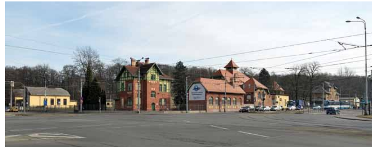
Fig. 5.1: Ostrava – water treatment plant, overall view. Photograph by Roman Polášek, 2019.
