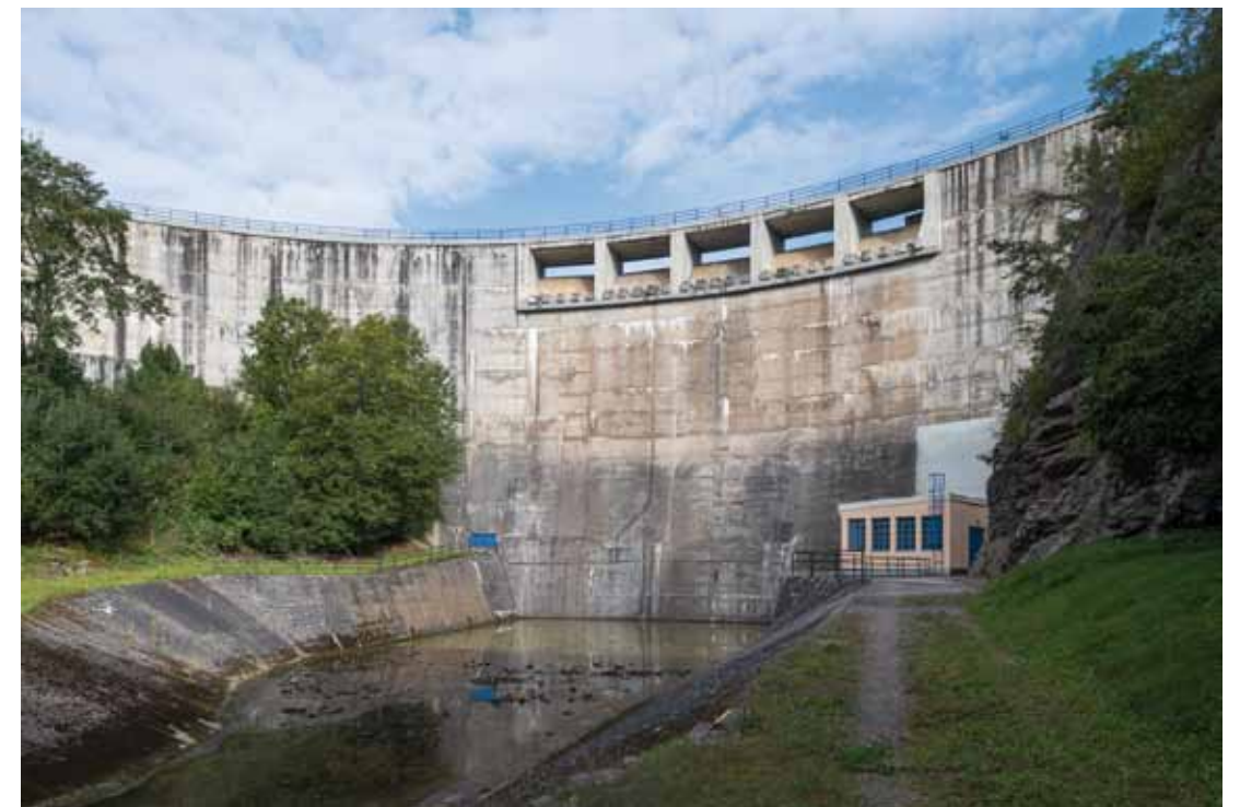
Fig. 4.21: The Vrchlice dam (1966–1970) – arch dam. Photograph by Viktor Mácha, 2020.
