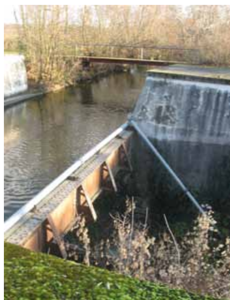
^ Fig. 4.92: The Semínský aqueduct on the Opatovice Canal: (A) state after reconstruction; (B) remains of old wooden elements. Photograph by David Honek, 2020.
