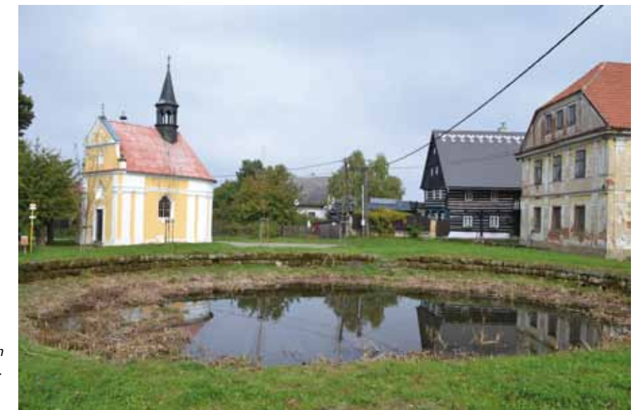
Fig. 4.46: Dražejov – reservoir in the middle of the village square, fed by rainfall and overflow from the local historical water supply. Photograph by Miroslav Kolka, 2014
