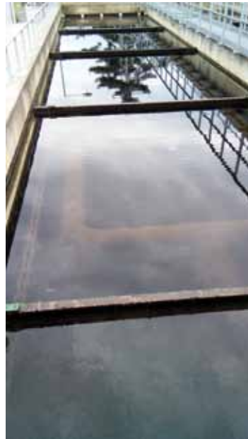
Fig. 4.243: Horizontal settling tank. Photograph from the TGM WRI archive.
