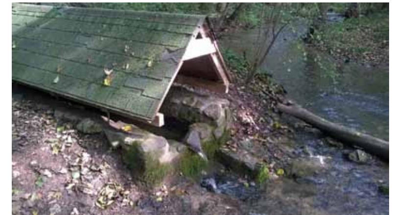
Fig. 4.207: Ochoz u Brna – spring tank (Kaprálova studánka) catching underground water springs in close proximity to the Říčka River. Photograph by David Honek, 2014.
