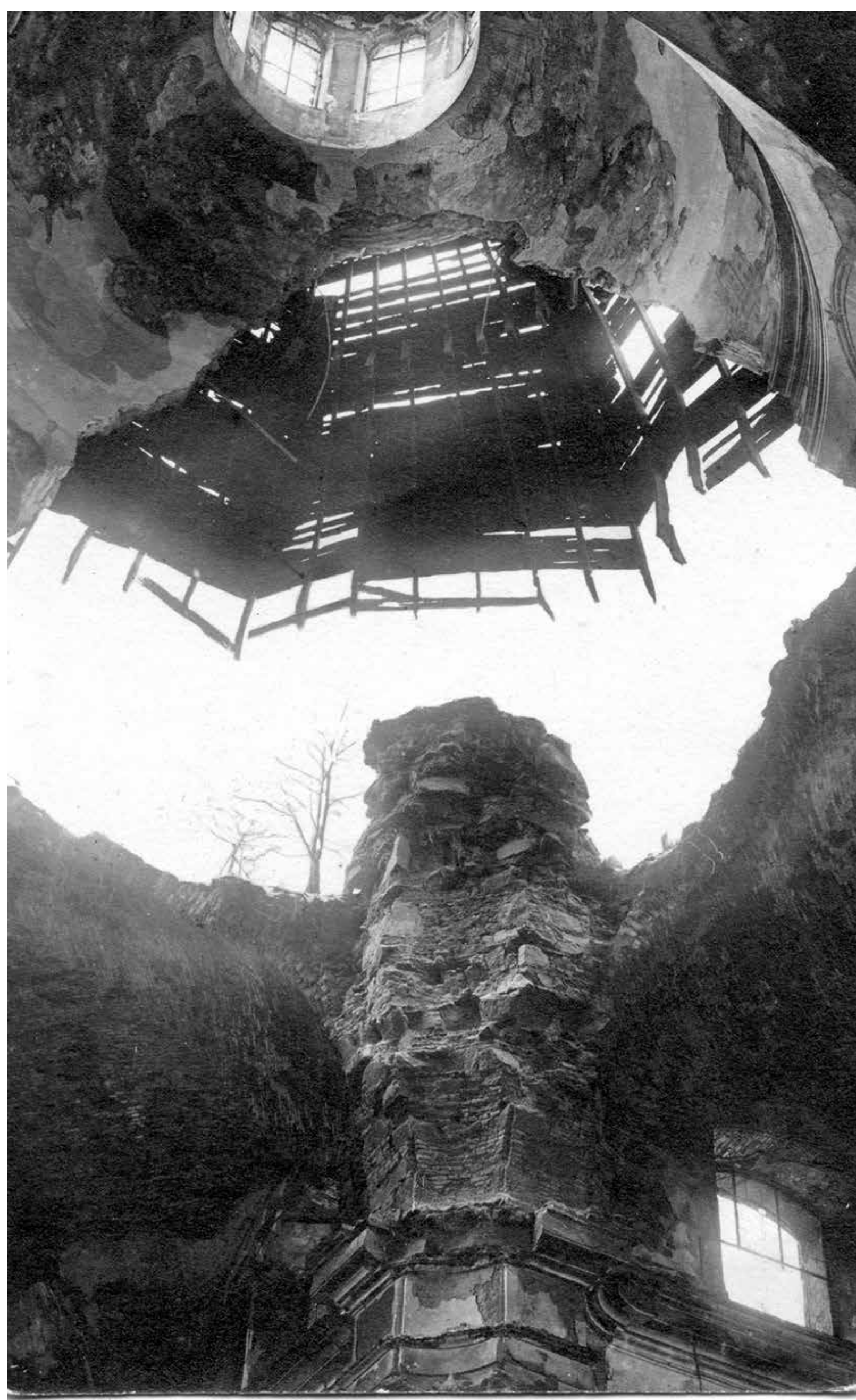
The church dome collapsed in 1920.
